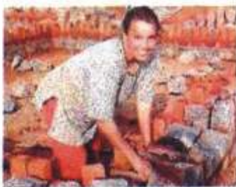
MUD IS THE WORD: Elke Cole uses cob, a mixture of sand, mud and straw to build houses.
